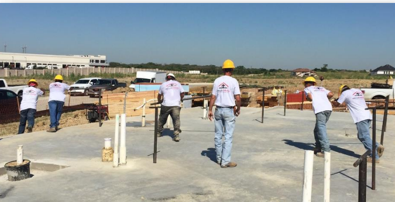
Tella Firma Crews Lifting the Foundation
